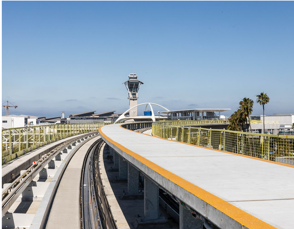
Guideway approaching CTA East Station
