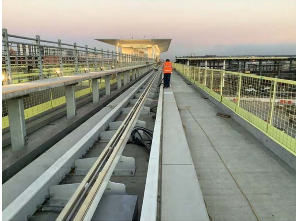
Guideway approaching ITFE Station
