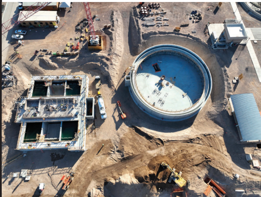
McCarthy ( No. 19 ) is CM-at-risk on the recently completed Kurt R. Segler Water Reclamation Facility Phase 4 Improvements project in Henderson, Nev. The project includes a new 12-million-gallon-per-day biological nutrient removal basin and a 125-ft secondary clarifier.
