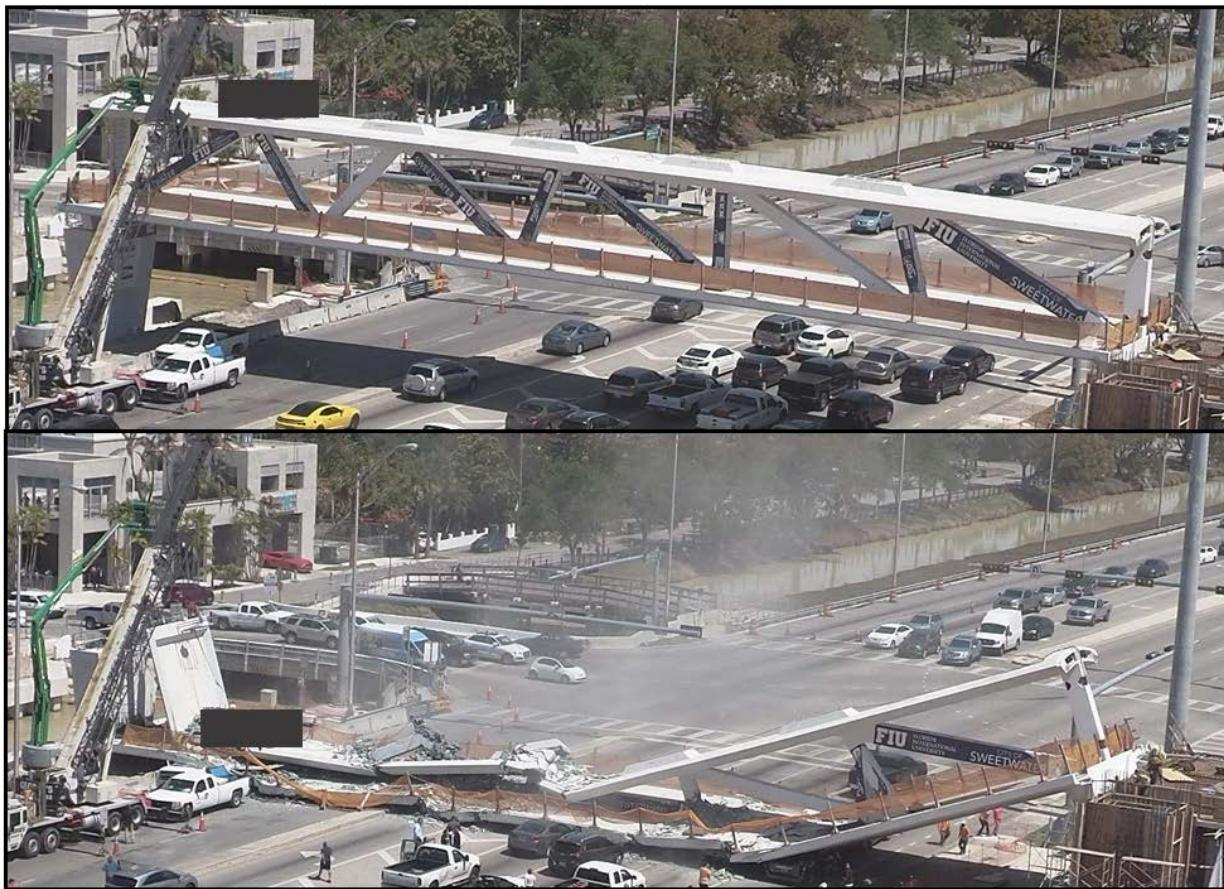
**Figure 4.** Still images from FIU parking garage camera, showing east views of pedestrian bridge, March 15, 2018, precollapse (top) and postcollapse (bottom). (Source: FIU video camera)
