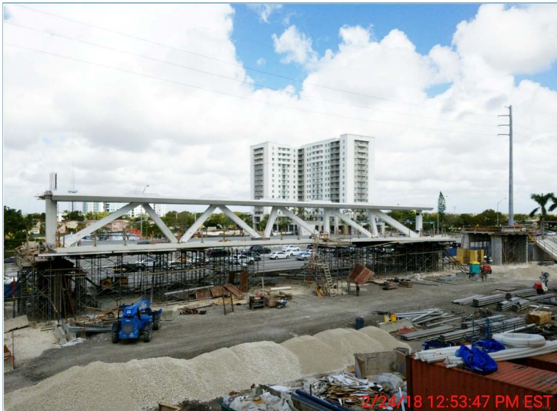
**Figure 15.** Temporary falsework supporting the bridge span in the casting yard on February 24, 2018, being sequentially removed from the middle of the span toward the ends of the span. (Source: MCM)
