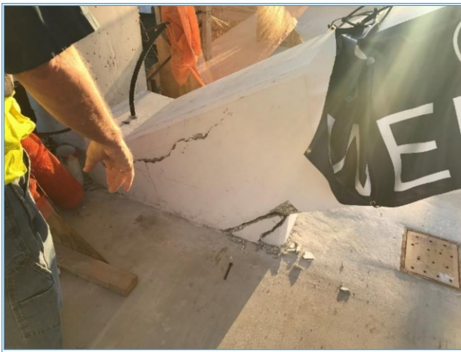
**Figure 25.** Cracks at bottom of diagonal member 11 (west view), March 15. (Source: FIGG)
