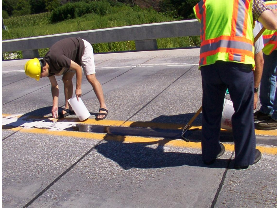
Figure 14. Application of Epoxy Coating and utility sand
