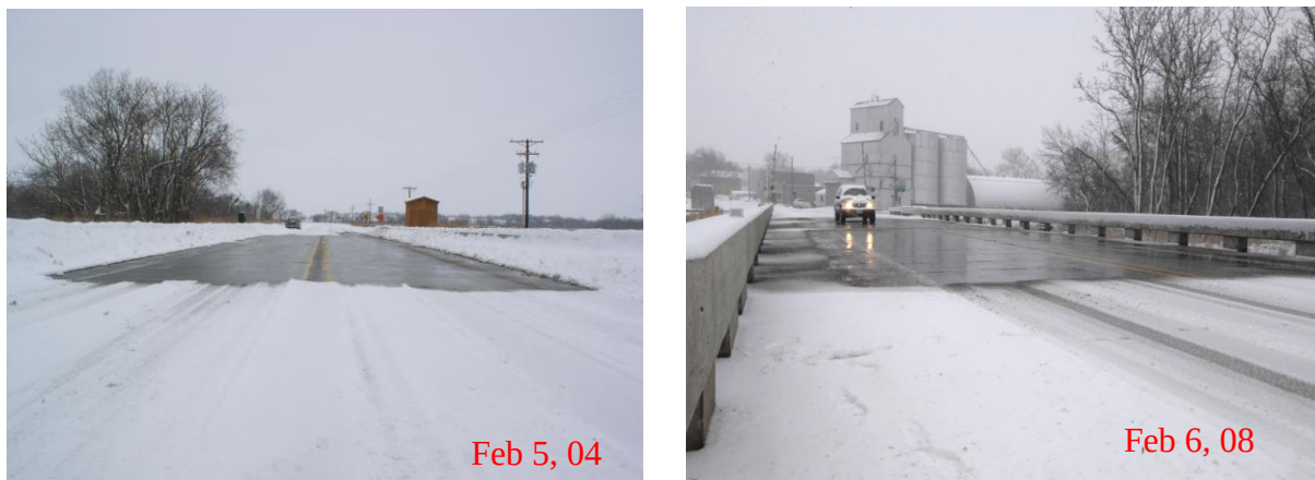
Figure 28. Roca Spur Bridge Deicing Operation
