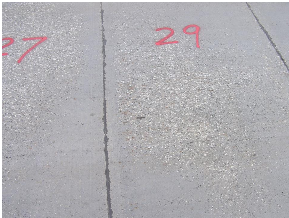
Figure 26. No Noticeable Deterioration in Westbound Lane Slabs
