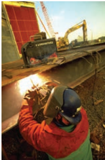
The portable wire feeder from Red-D-Arc does not require a control cable.
